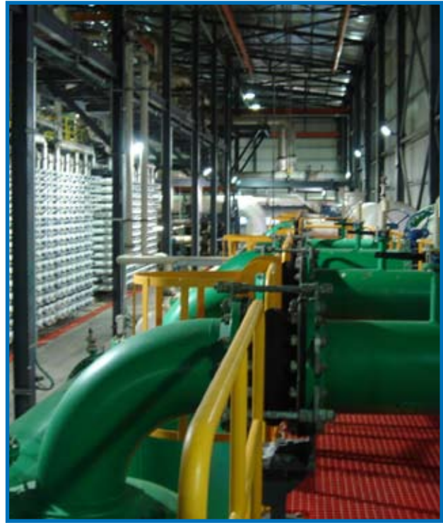
The IDE 330 ML/day Ashkelon Plant, Israel, is the world's largest reverse osmosis plant
