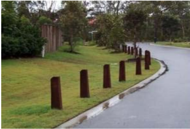
Grassed swales incorporated into residential streets in Brisbane
