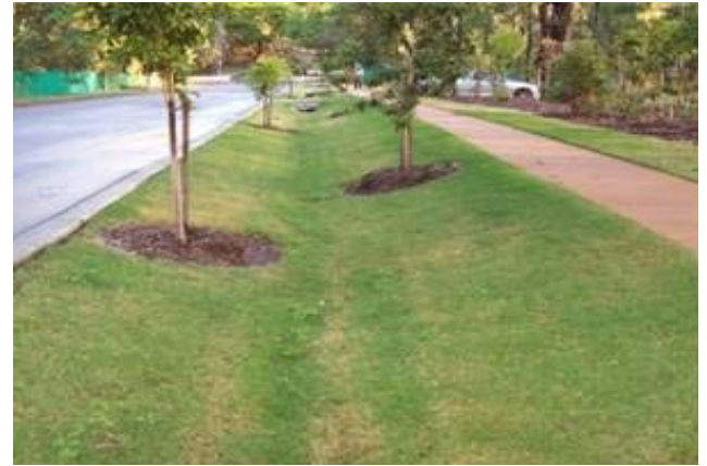
Grassed swales incorporated into residential streets in Brisbane
