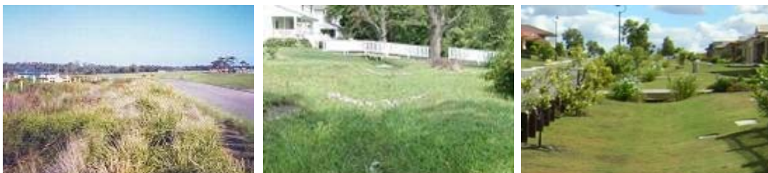
Plate 13.3-B: Swale systems: heavily vegetated (left), use of check dams (centre), grass swale with elevated crossings (right)
