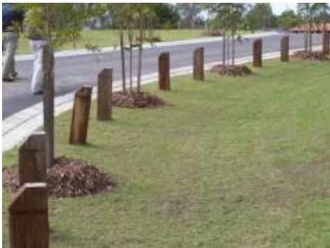
Plate 13.3-H: Traffic bollards mixed with street trees to protect swale from vehicles
