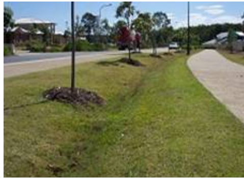
Plate 13.3-D: Swale located in road reserve
