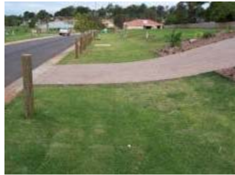
Plate 13.3-A: Typical swale profile in residential street (trees to substitute bollards as traffic controls)
