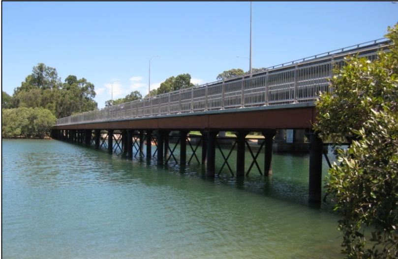
Currumbin Creek Railway Bridge, 2017. Image courtesy of City of Gold Coast.
