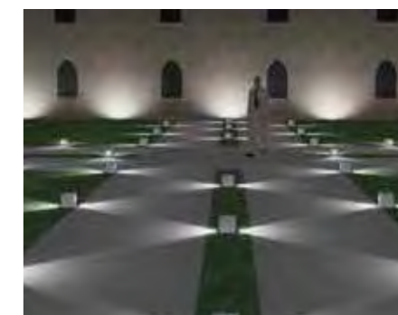
(PL 1) GROUND MOUNTED LED BOLLARDS
