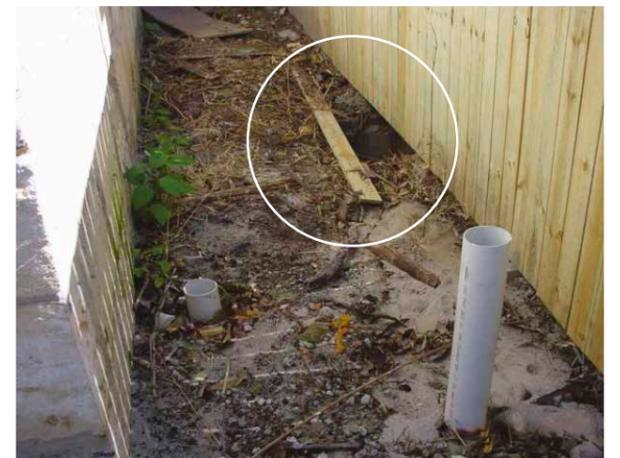
Structures, including fences, should be clear of field gully inlets. Suitable landscaping along with grid tops to inlets and regular maintenance assists with filtration into the City's stormwater system.
