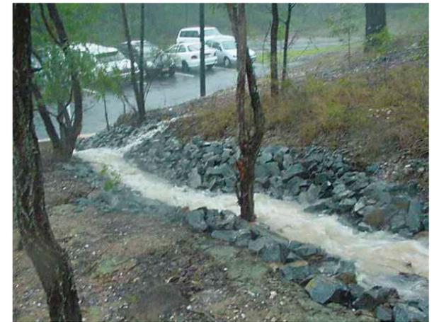
Diversion drains can assist to drain water away from buildings and level areas on sloping properties.
