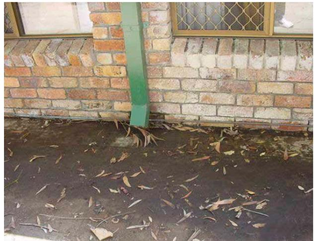
Roof guttering not connected to approved stormwater outlets can cause damage to your property and neighbouring properties.
