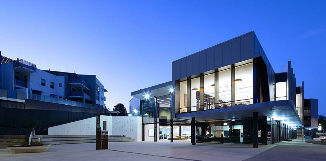
Photograph 6.2.154-1 Example of a Community use located at Helensvale. Photograph by John Mills.
