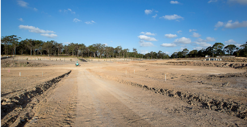
Photograph 9.4.1-1 Example of changes to ground level and creation of new waterways located at Coomera. Photograph by Remco Jansen.
