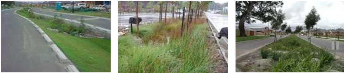
Plate 13.0-B: Bioretention Swales are commonly located in median strips of roads and carparks
