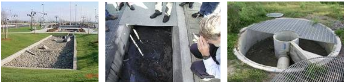
Plate 13.0-G: Sand Filters can be installed above or below ground
