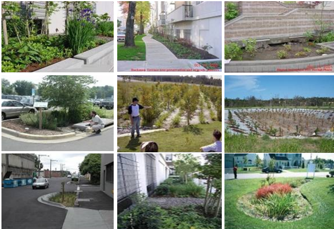
Plate 13.0-D: Bioretention Basins are applicable at a range of scales and can be integrated into an urban landscape
