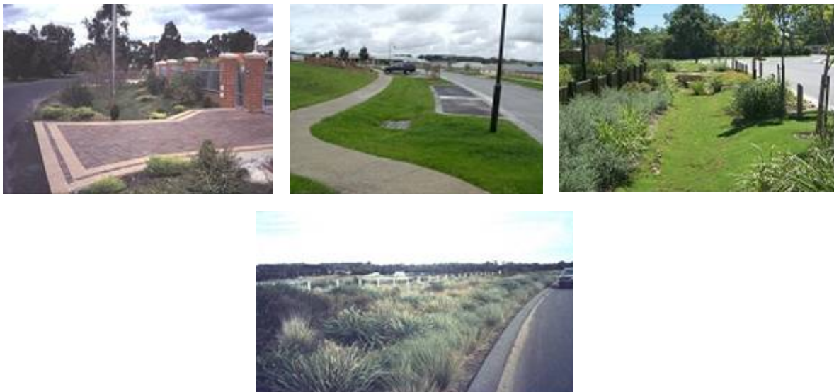
Plate 13.0-A: Swale Vegetation is selected based on required treatment performance and appearance
