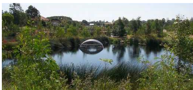
Figure 13.5-F: Top: Example Layout of Sedimentation Basin ‘Control’ Overflow Pit and Pipe Connection to a Macrophyte Zone. Bottom: Control Overflow Pit Installation
