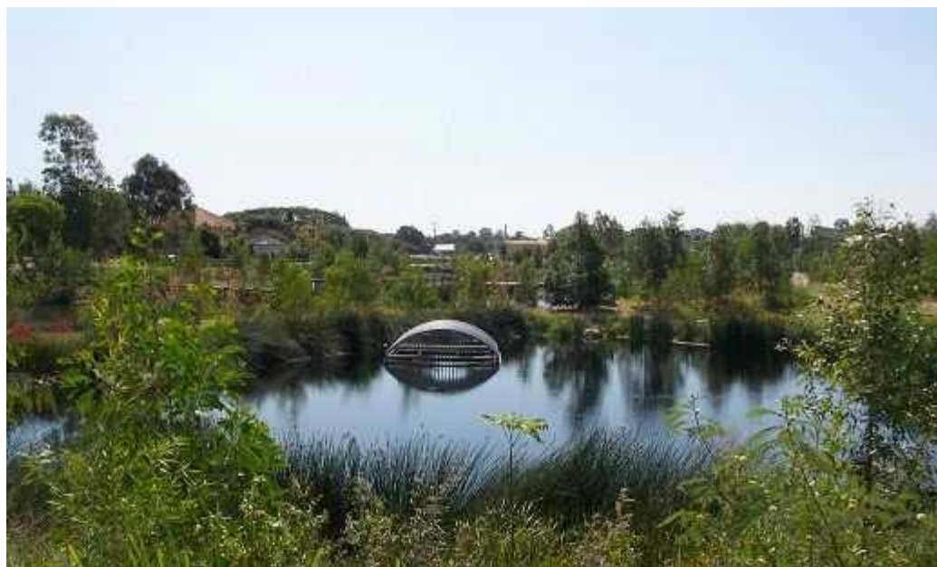
Sedimentation Basin as an inlet zone for a constructed wetland in Brisbane
