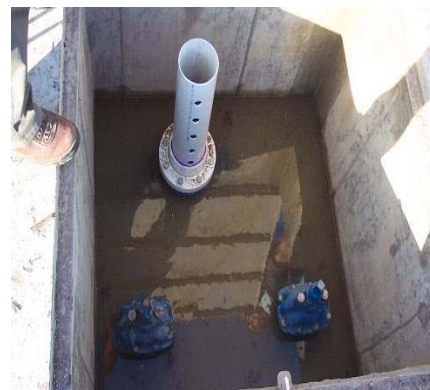
Plate 13.7-E: Macrophyte Zone Outlet Arrangement
