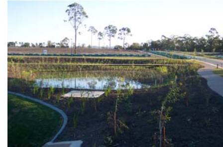
Plate 13.7-H: Constructed wetland functional installation
