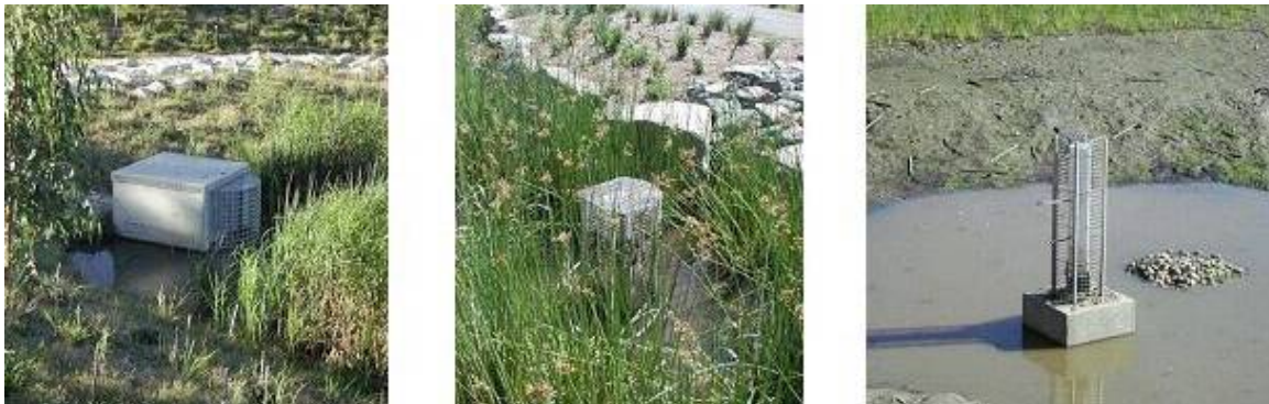
Plate 13.7-D: Example Outlet Riser Assemblies with Debris Guards
