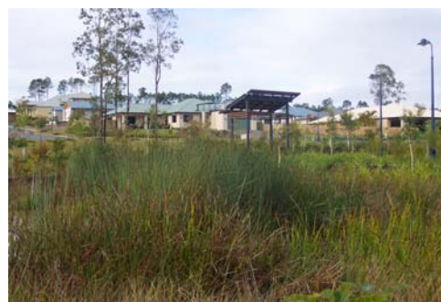
Plate 13.7-J: Constructed wetland operation establishment
