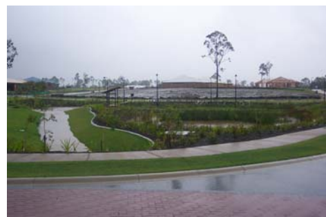
Plate 13.7-I: Constructed wetland sediment and erosion control
