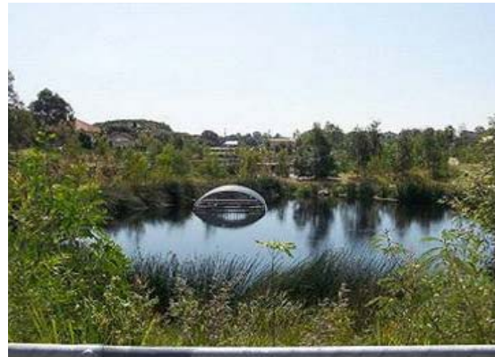
Plate 13.7-B: Inlet zone of a constructed wetland in Brisbane
