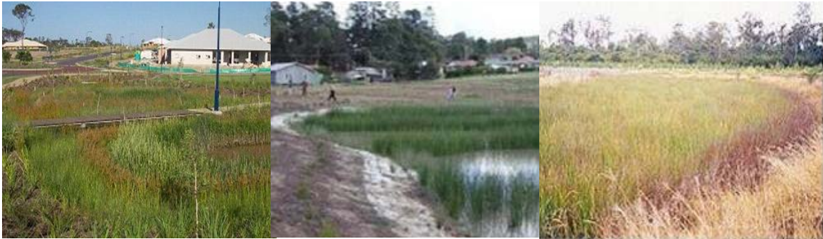
Plate 13.7-C: Macrophyte zone planting and bathymetry
